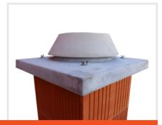
10. Clean the modified cut chimney liner block, apply joint compound on it and fit the chimney collar. Wipe off the excessive joint compound and clean the joint. A gap of 15 mm should remain between the top edge of the covering plate and the bottom edge of the collar for chimney ventilation.
