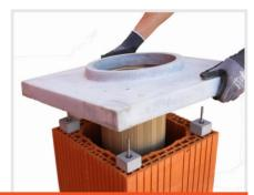
9. Insert the screws of the fixing set (HSU, if no reinforcement has been used) into all corners of the last chimney block (HU) and pour grout into the holes. Put the spacers (HDP) on the screws. Drill holes in the cover plate with a drill without hammering according to the dimensions of the inserted screws. Fit the cover plate and carefully tighten the wing nuts to prevent the screws from being torn out.
